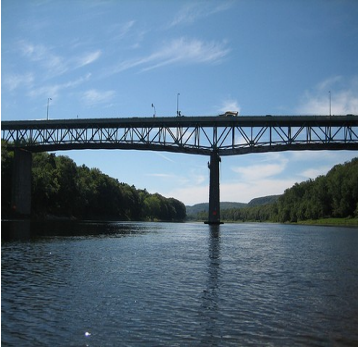
An additional five feet of depth would give the Delaware the capacity for larger cargo ships to come through the ports
